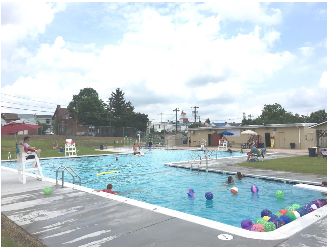
Figure 1: Emmitsburg Community Pool as of June 2018 (newly renovated in 2018).
